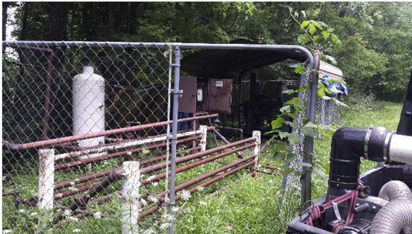
Fig. 3. Site 3 was an out of service gathering station with a significant number of leaking components. The FFS system, mounted in the back of the UTV, can be seen in the bottom right corner of the figure.
