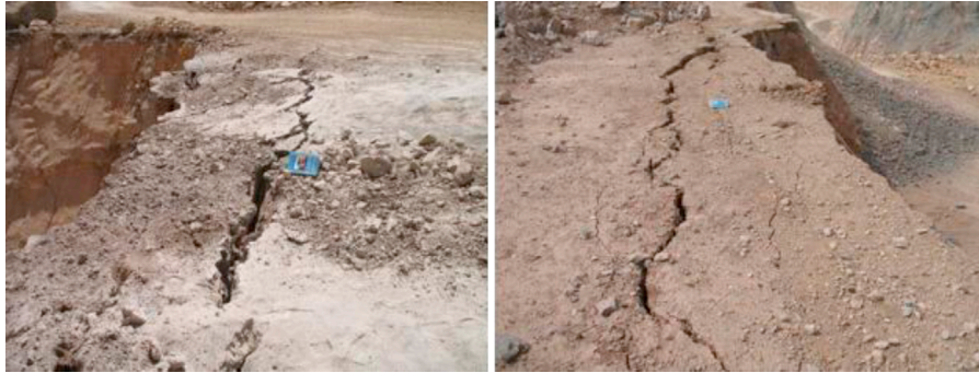
Fig. 2. The undesirable backbreak after blasting in mines.
