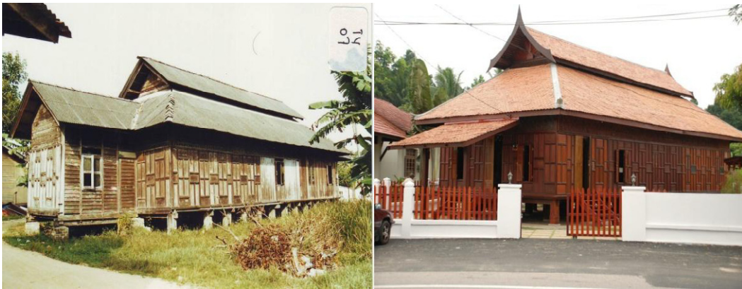
Figure 3: Kedai Mulong Mosque, before and after restoration (2009). The original buildings (left) was a palace hall ( balai istana ) and located at Kota Bharu, in 1958 have been relocated to Kedai Mulong. The restoration of old mosque was based on historical and physical documentation. The new mosque is compatible with the historic/original character of palace hall.
