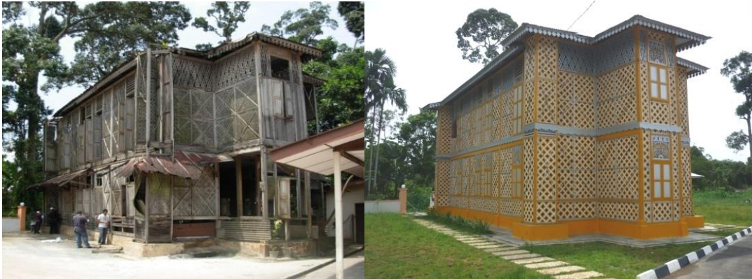
Figure 1: Kampung Kuala Dal Old Mosque, Kuala Kangsar (before and after conservation, 2009). The conservation of this mosque achieves the aims of heritage conservation. The plaited bamboo walls and carvings was restored base on original form, design and materials. The wall's panel also been paint base on original colour schemes.
