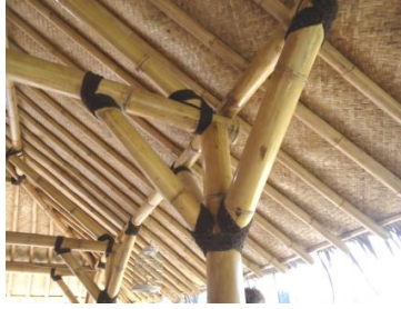
Fig. 2. Example of traditional bamboo jointing method – Natural fibre rope “ijuk”.
