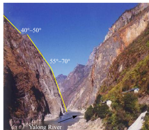
Fig.12 A deeply cut V-shaped valley at the dam site of Jinping I hydropower station.
