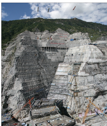
Fig.21 Overview of the left bank slope after excavation.
