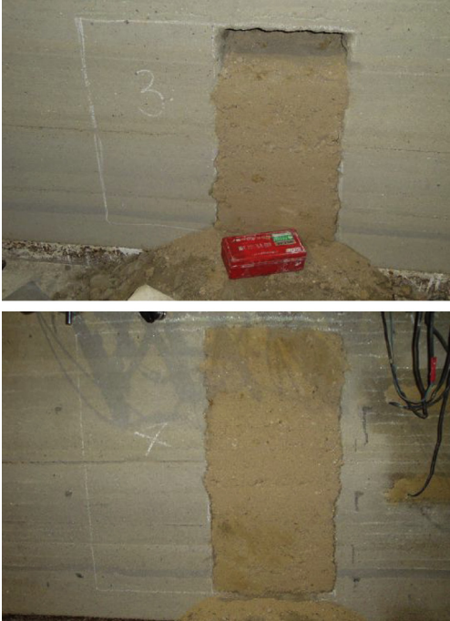
Fig. 7. Backfilling the primary room with cemented material.
