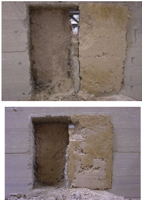
Fig. 8. Extracting ore to form secondary room.
