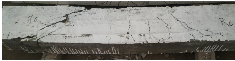
Figure 11 Crack pattern at failure of high strength RC beams with stirrups.
