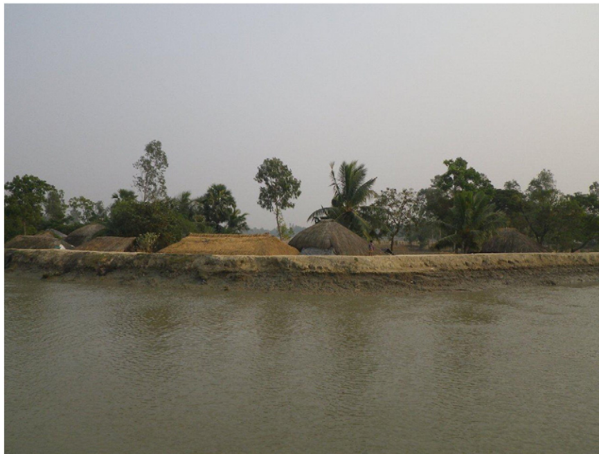
Fig. 4. Subsidence and reduced sedimentation due to embankment construction has led to river levels being higher than adjacent land levels in the Sundarbans, West Bengal, India, reinforcing that subsidence can have local causes. Courtesy of Attila Lázár (taken January 2014).
