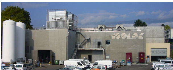
Fig. 1. Picture of the ISOLDE facility with the new buildings that host the compressor, and the cold box of the new superconducting HIE-ISOLDE linac.
