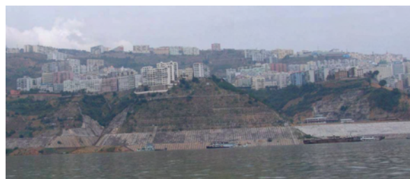
Fig.17 Overview of Yuhuangge landslide and densely relocated buildings.
