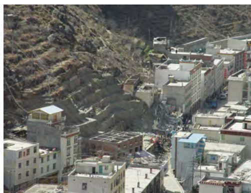
Fig.10 Reactivated landslide due to irrational slope cutting (2003).
