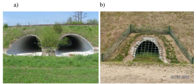
Fig. 3. Underpasses: (a) for small animals; (b) for amphibians.
