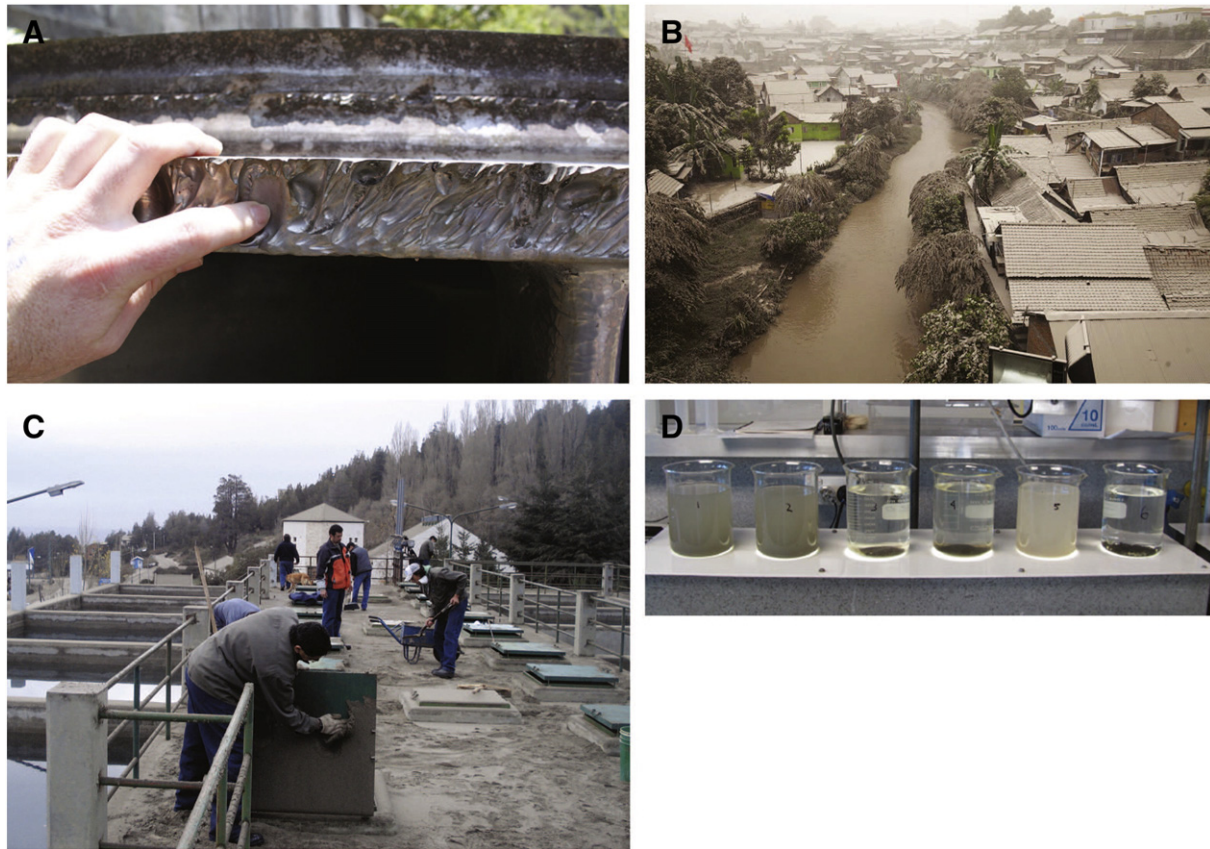
Fig. 6. (A) Abrasion damage to a turbine removed from the Agoyan hydro electric power station, Ecuador as a result of exposure to tephra laden water derived from the 1999–2010 eruptions of Volcán Tungurahua (photo: Johnny Wardman). (B) Houses covered with a thin layer of tephra after the eruption of Mt. Kelud on February 14, 2014 (photo: Dwi Oblo). (C) personnel cleaning tephra from the Bariloche, Argentina water treatment plant after the June 4, 2011 eruption of PCCVC (photo: Carol Stewart). (D) Laboratory experiments to determine the settling rate of tephra in water. Each beaker contains a different tephra and shows the turbidity after 1 h of settling (photo: J White).
