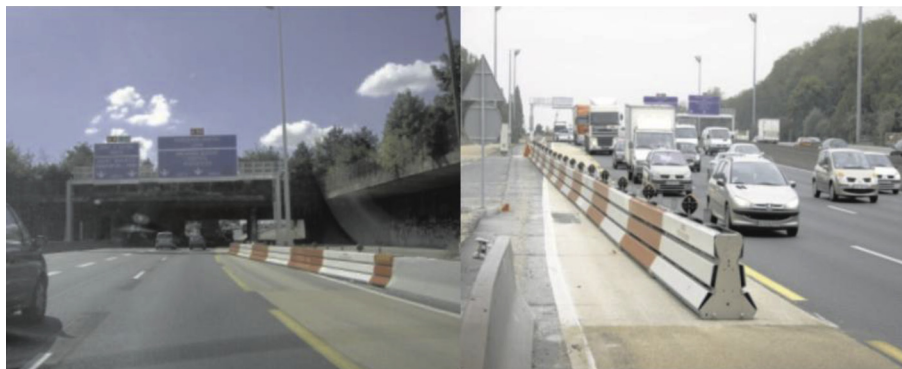
Fig. 2 – Weaving A4-A86 section, eastbound with 5th lane, open and closed.
