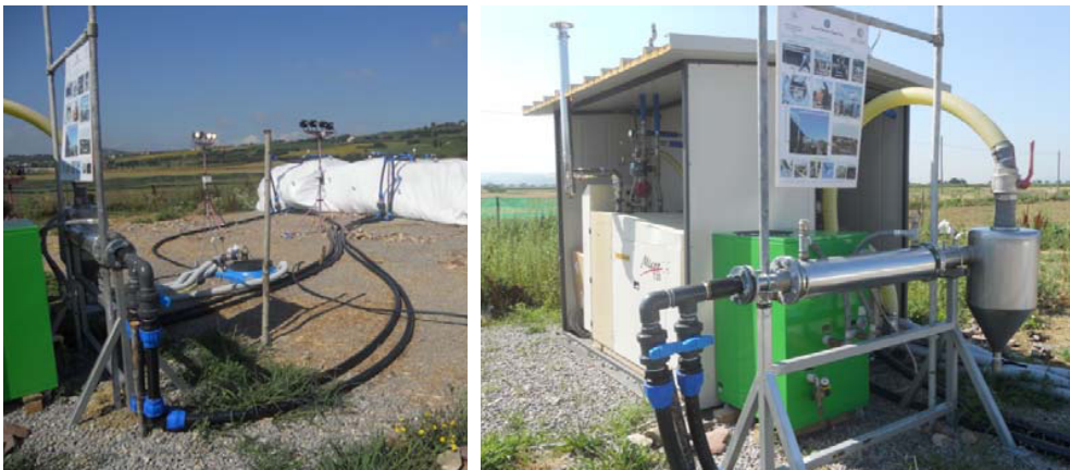
Fig. 1. (a) The biocells as biomass digester; (b) Dehumidification unit and 30 kW powered CHP engine.
