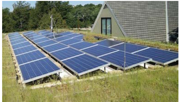
Figure 2: Center for Design Research (CDR) Roof
