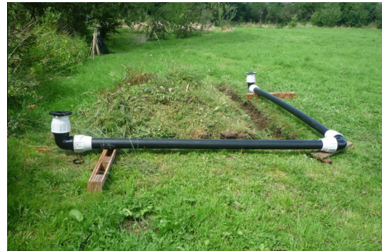
Fig. 4. Pipe rig just prior to burial.
