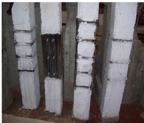
Fig. 2 R.C columns after jacketing.
