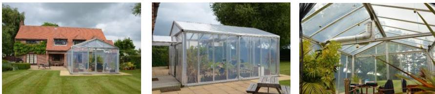
Fig. 2. The external and internal views of the Test Structure with ETFE encapsulated panels
