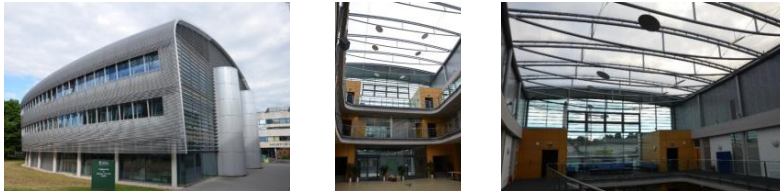
Fig. 1. The external and internal views of the ESLC Building
