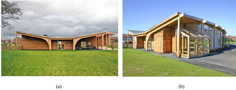
Fig. 2. (a) Kingsmead School Elevation; (b) Wooden Surfaces and Details
