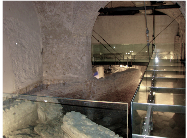
Figure 14 Palazzo Valentini, domus: suspended footbridges with transparent floors and parapets.
