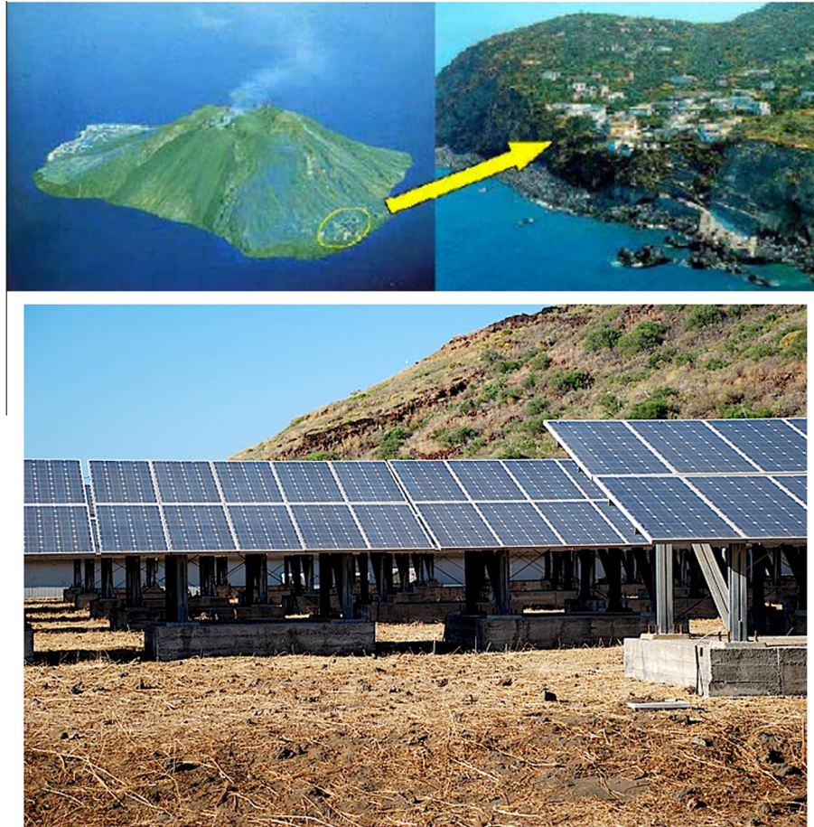
Figure 2. 100 kW photovoltaic field in Ginostra, an isolated fraction in the island of Stromboli, Sicily, now electrified with a hybrid PV-diesel system powering also a desalination plant.
