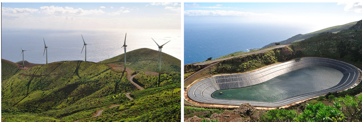
Figure 6. Five wind turbines (left) coupled to an hydroelectric plant using an artificial basin at the bottom of the extinct volcano (right) and the volcano's crater, now provide almost the whole energy needs of El Hierro island, in the Canaries archipelago. [Reproduced from technocrazed.com, with kind permission.]
