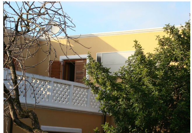
Figure 8. Sicily’s home heated with solar air. Relative humidity went from >80% to an average 55% in less than 4 days. Since then, the home has never suffered from high relative humidity again. [Photograph of Mario Pecoraino.]
