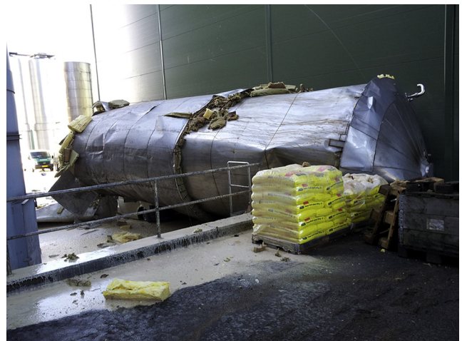
Fig. 2. The van is visible under the tank. The tank contents washed up on the elevated platform. (Photo courtesy of the company.)
