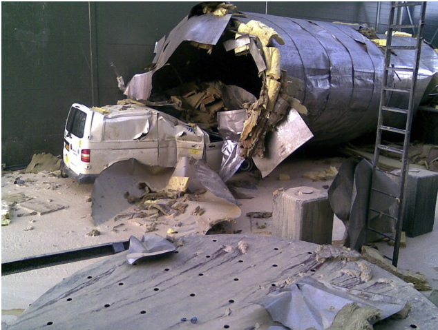
Fig. 3. The tank landed on the van and crushed it. The tank's original position (the sloping support structure for the tank floor plate) is in the foreground. The tank floor plate is center left. (Photo courtesy of I.W. Michaelsen.)
