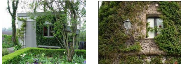
Fig. 2. Vines are encroaching on windows (left) and the remnant traces of climbers on residences (right).
