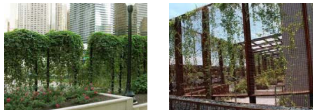
Fig. 4. Freestanding fence mounted upon trellis column supports
