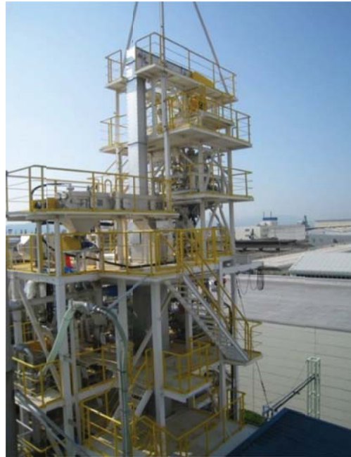
Fig. 4. Appearance of the KCC moving-bed bench-test plants.
