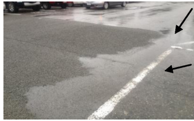
Photo 12. Run-off being captured by pervious concrete.
