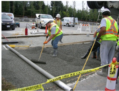
Photo 6. Roller screed and leveling of pervious concrete.
