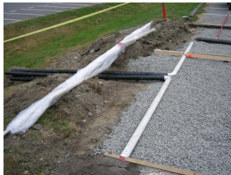
Photo 2. Perforated pipes on top of crush connecting to ABS pipes.
