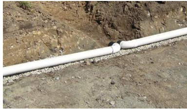
Photo 1. Perforated pipes above the subgrade.
