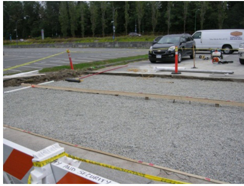
Photo 5. Compacted crush ready to receive pervious concrete.
