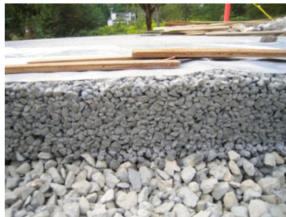
Photo 9. Pervious concrete cross-section after saw cut.
