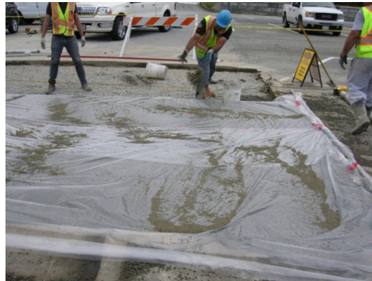
Photo 8. Finished concrete slab (Bay 1) covered with polyethylene sheet.
