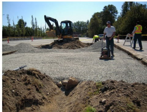
Photo 4. Compaction of clear crush and simultaneous excavation.
