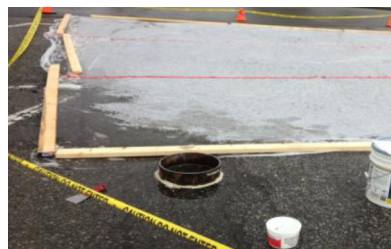
Photo 11. Ring used for the in-place percolation test.
