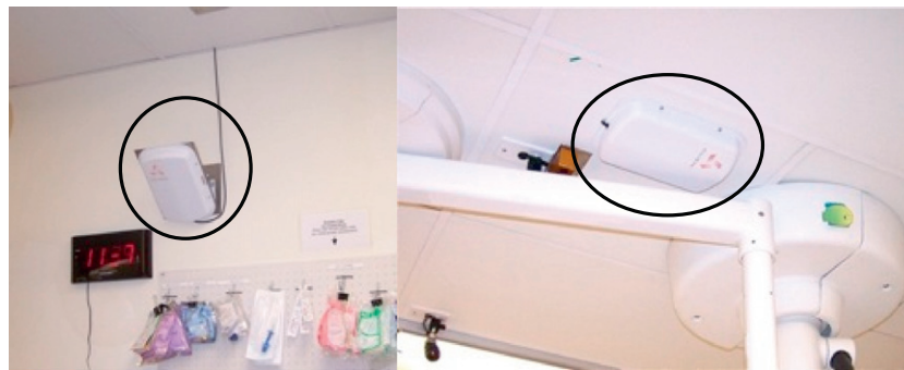
Fig. 5. Positioning of angled and ceiling-mounted antennas at CNMC. Left picture shows angled antenna #1. Right picture shows ceiling-mounted antenna #3.
