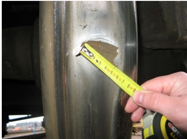
Fig. 7. Crack length measuring with a ruler.
