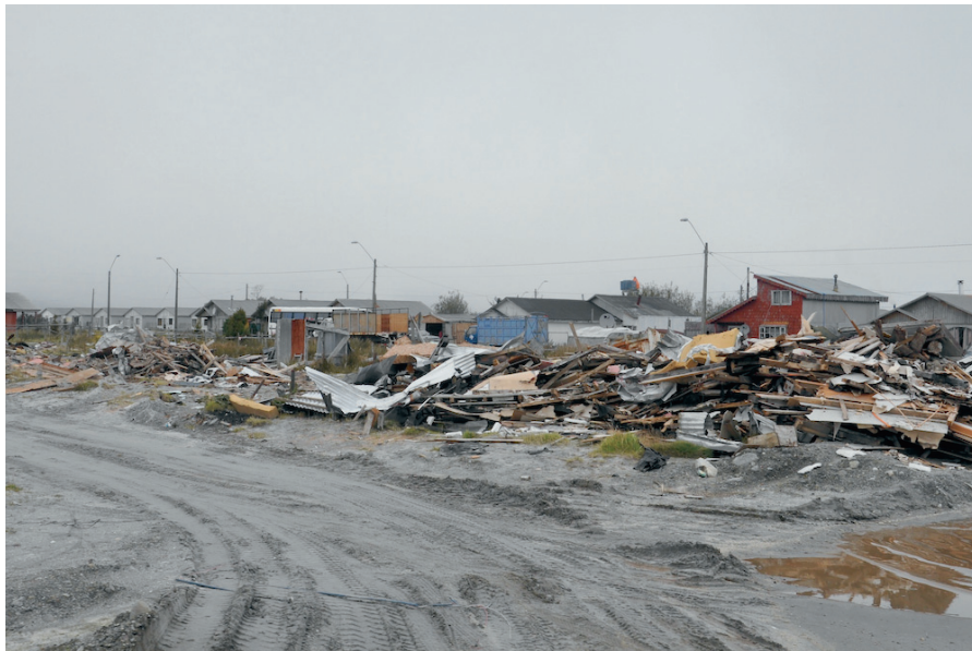
Fig. 3 Part of demolished housing units in southern Chaiten
