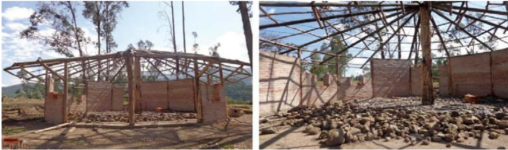
Fig.5. Chapel exterior view, Chapel interior view
