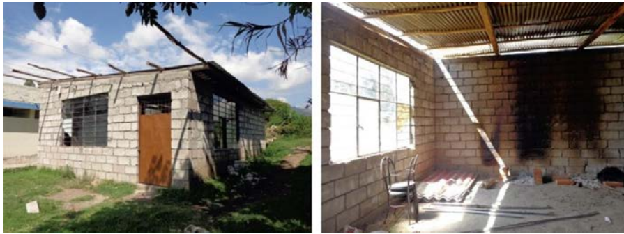
Fig.8. Kitchen external view, Kitchen internal view
