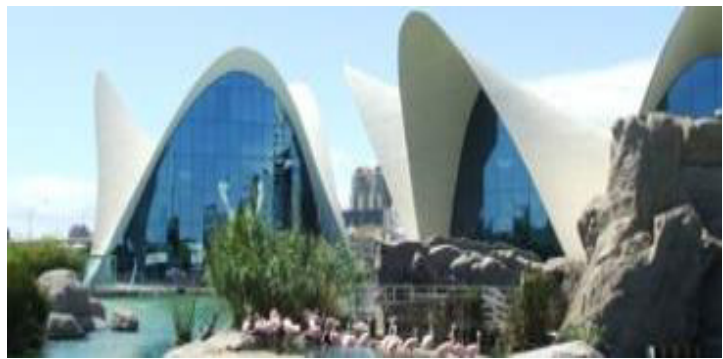
Fig. 3: SFRC shells made in the European Oceanographic Park in Valencia [2]
