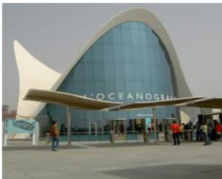
Fig. 2: SFRC shells made in the European Oceanographic Park in Valencia [2]
