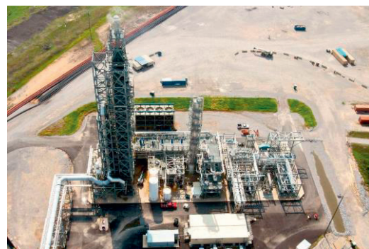
Fig. 2 Aerial Photo of the Capture Plant
