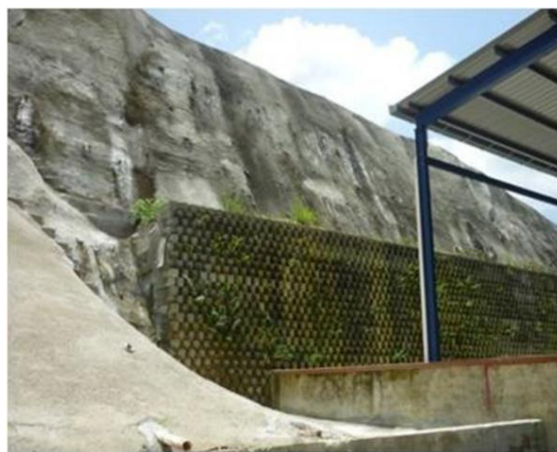
Fig. 5. Slope face after stabilization [3]
