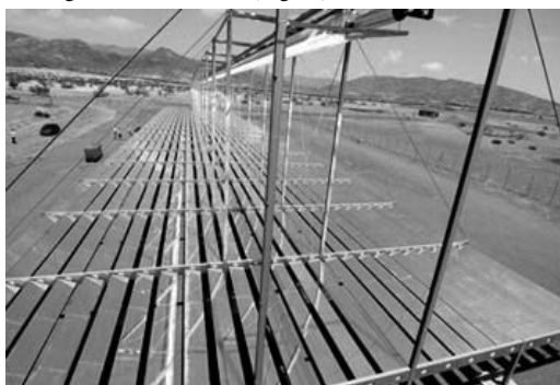
Fig. 3. Line focusing, linear Fresnel reflector: The solar mirror Fresnel Almeria in Andalusia (Spain)
