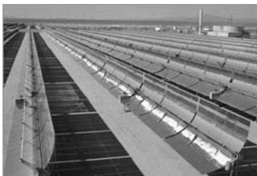
Fig. 2. Line focusing, parabolic trough collector: The solar parabolic trough mirror Hassi Rmel (Algeria)
