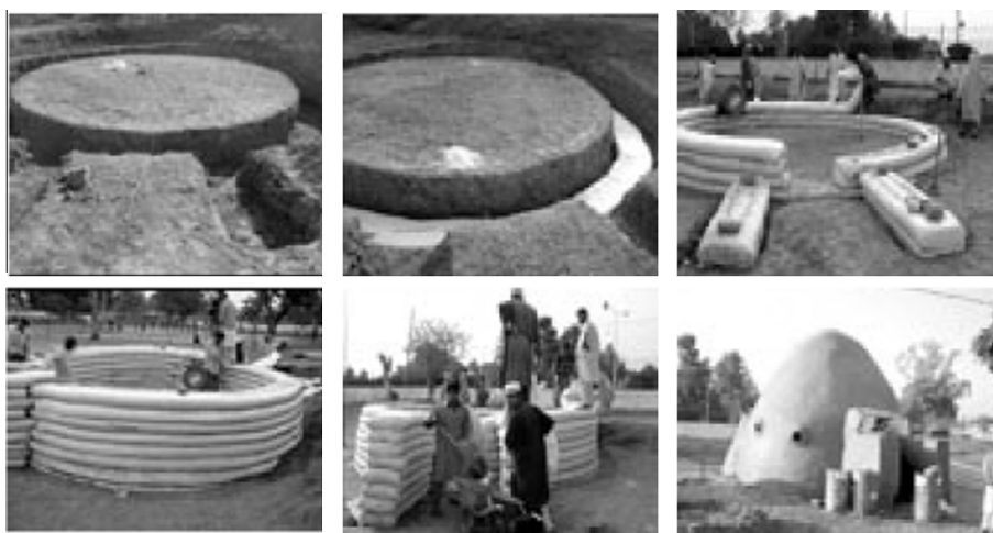
Fig. 4 The 'superadobe' houses construction sequence ( http://calearth.org/building-designs/emergency-sandbag-shelter.htm : accessed on 20th of April 2013).
