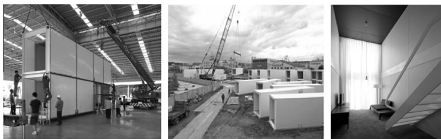
Fig. 6 (Left) The complete assembly of the 'EX-container' in factories. (Middle) The deployment of the 'EX -container' in sites. (Right) An interior view of the 'Ex-container' ( http://exc.ysmr.com/container_e/ : accessed on the 21st of April 2013).
