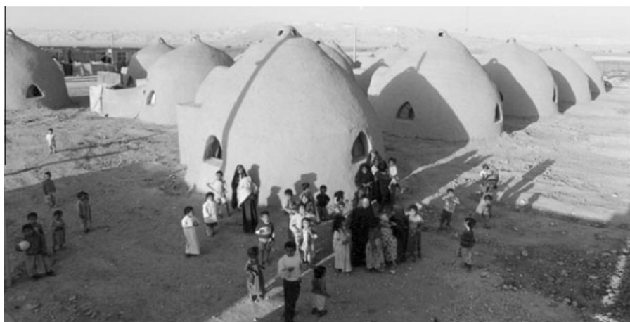
Fig. 5 The 'superadobe' domes with their streamlined form ( http://calearth.org/building-designs/emergency-sandbag-shelter.htm accessed on 20th of April 2013).
