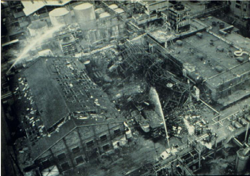
Fig. 3. Plant destroyed by a rupture of a batch reactor, 1969 [11].
