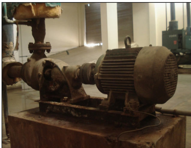
Fig. 1. 2.1 HP motor used for dearator transfer pump.
