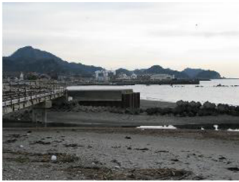
Fig. 15. Photograph of left bank jetty taken from right bank of river mouth.
