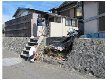
Fig. 10. Rusted winch left in gap of seawall.
