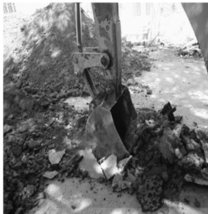
Fig. 3 Excavator bucket working during field test
