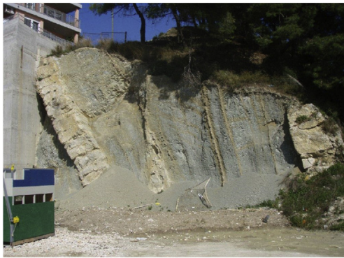
(e) Second phase of protective structure completed (2010).
