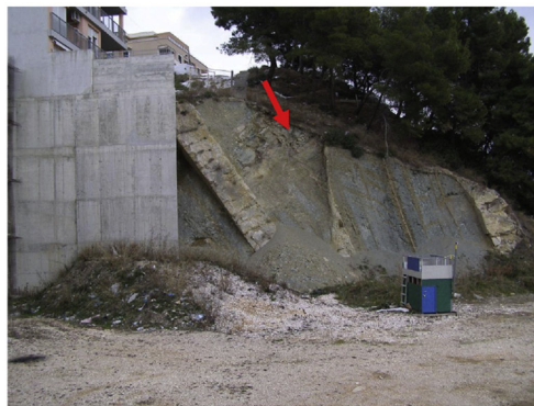
(g) Material fall at cut slope (2012).
