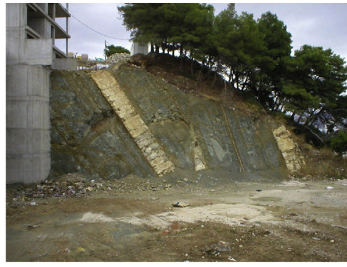
(b) First phase of protective structure completed (2004).
