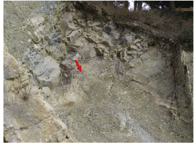
Fig. 13. Sliding along secondary joint set.
