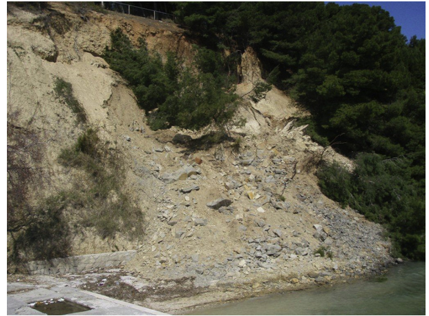
Fig. 3. Landslide along the coastal cliff in flysch formation (Duilovo, Split).
