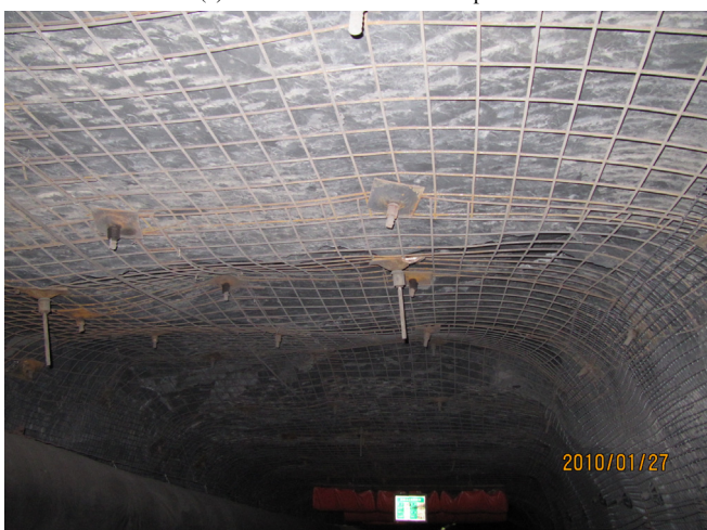
(b) Roadway roof.
