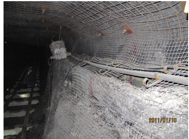
(a) Overall outward movement of sidewall in the narrow coal pillar.
