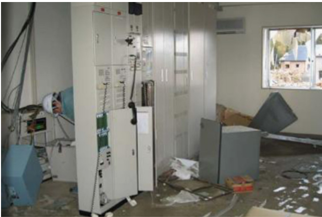
Photo 1. Data logger of KSN Station which was damaged by the tsunami.
