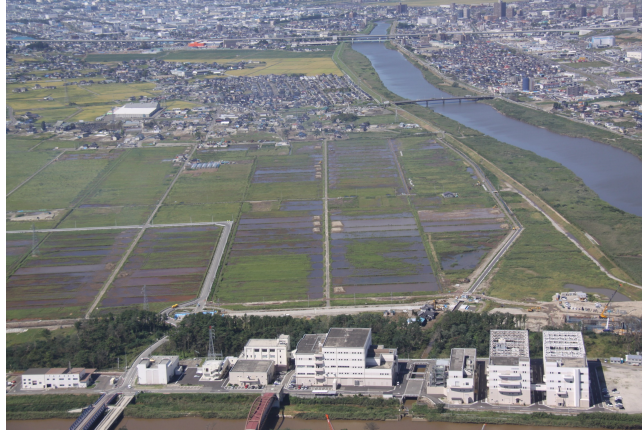
Figure 1(b). An aerial view of purification center used for photogrammetry surveys
