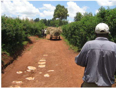
Photo 8. Exposed “do-nou” at slope.
