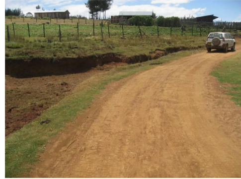
Photo 7. Road conditions at same place shown in Photo 6 after maintenance in Kenya.
