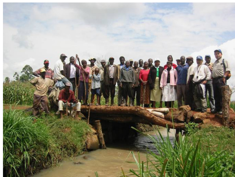
Photo 9. Log bridge constructed after demonstration of “do-nou”.
