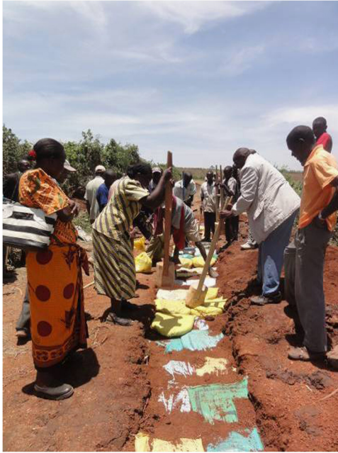
Photo 5. Communities compacting “do-nou” for road maintenance in Kenya.
