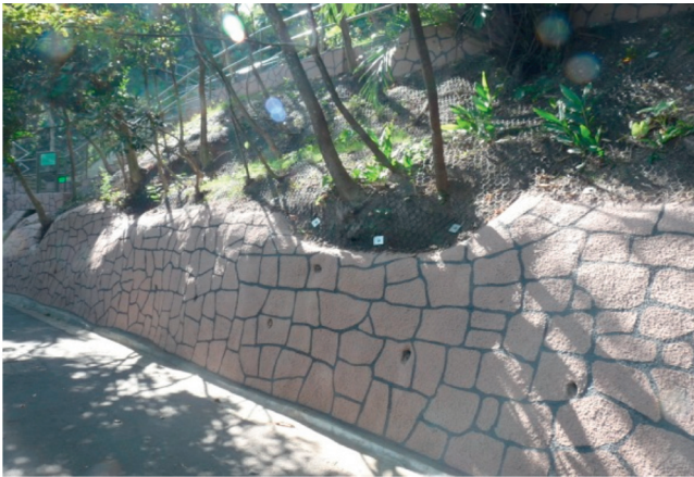
(a) Masonry-like finish on hard slope cover.
