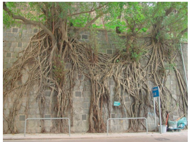
(b) Soil nails on an old masonry wall.
