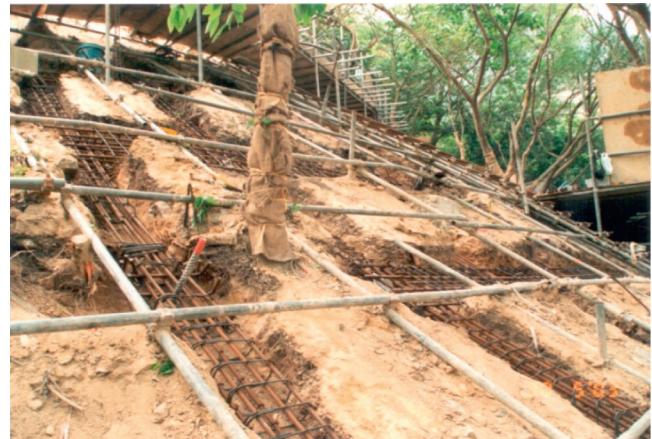
(a) Construction of soil nails and grillage.
