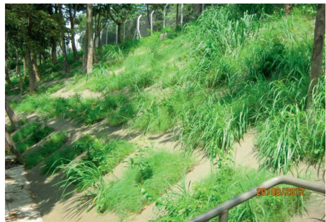
(b) Completion of soil nails and grillage construction.
