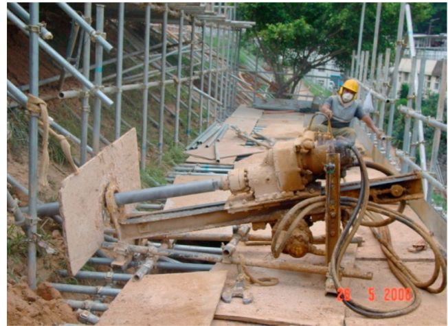
(a) Construction of soil nails in a soil cut slope.
