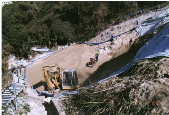
(a) Re-compaction of existing fill.
