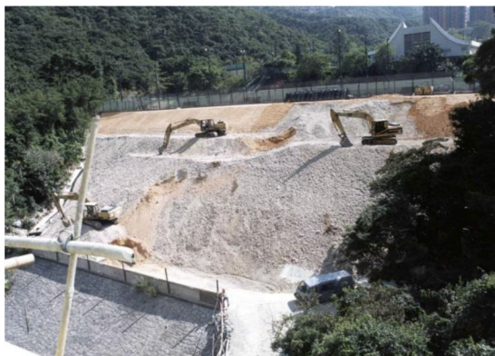
(b) Application of rock fill cap.
