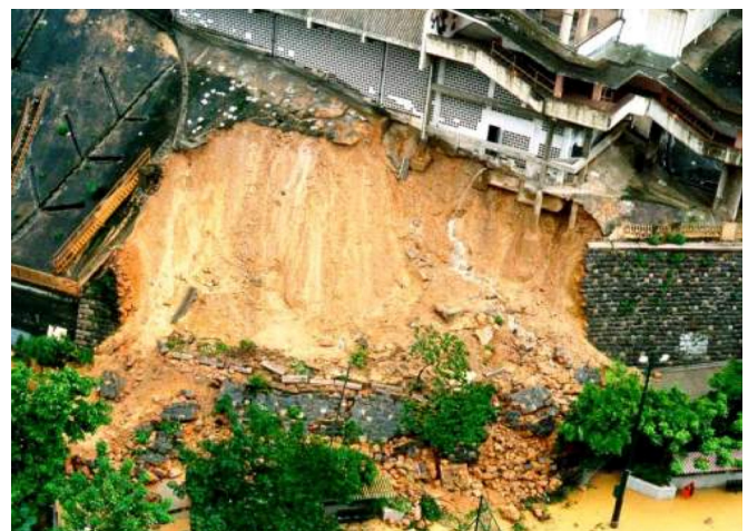
Fig. 6. The 1994 fatal landslide at Kwun Lung Lau.
