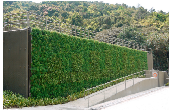
(a) Vertical greening on a concrete barrier.
