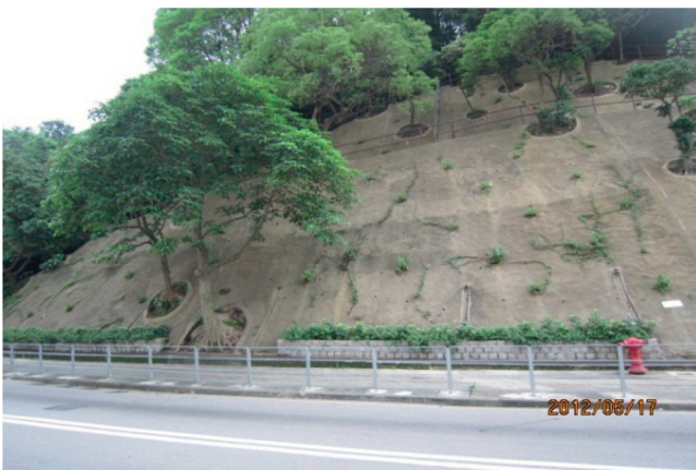
(b) Provision of planter holes and toe planter.
