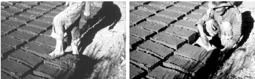
Fig. 1. Typical moulding technique of Adobe bricks ([13,14], 63).
