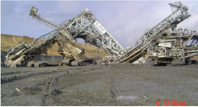
Fig. 1. Collapse of bucket wheel excavator SRs 1760 [10]
