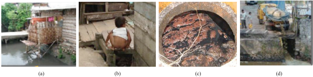
Fig. 1. Poor sanitary condition in Indonesia; (a) Poor quality latrine; (b) improper faeces disposal; (c) septic tank leakage and; (d) illegally sludge dumping [6]
