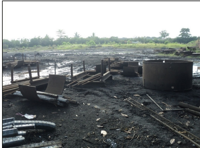
Figure 1. First work station
