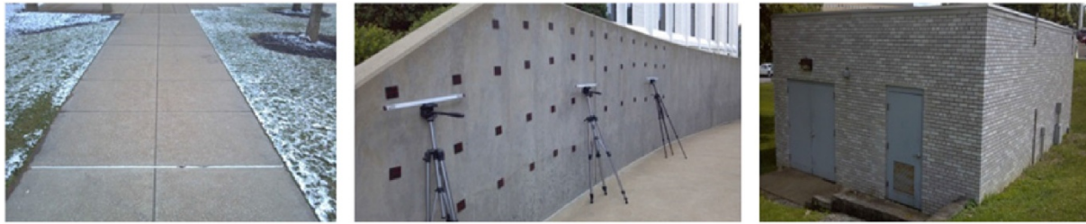
Figure 8 Left to right: sidewalk slab, retaining wall, and storage building.
