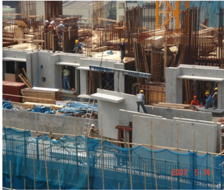
Figure 1 Precast façade installation on site.
