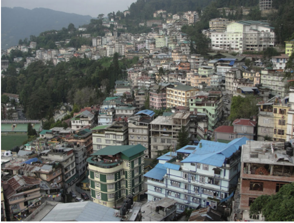
Fig. 63 Dense, unregulated reinforced concrete frame construction on slopes in Gangtok city, located in seismic zone IV (photo: C. V. R. Murty)
