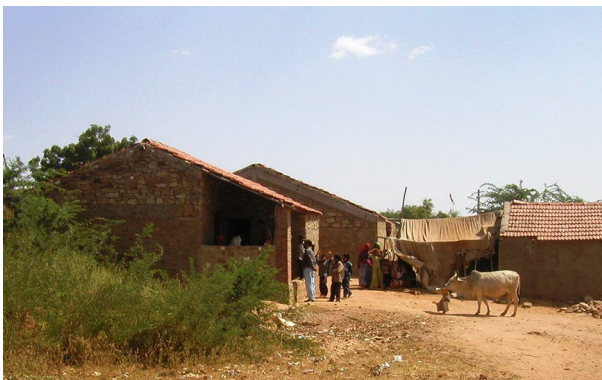
Fig. 45 Owner driven housing reconstruction after the 2001 Bhuj earthquake (photo: C. V. R. Murty)
