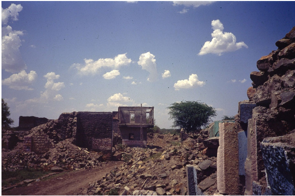
Fig. 38 Typical destroyed village in 1993 Latur earthquake (photo: S. Brzev)
