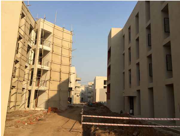
Fig. 57 Same student hostels, nearing completion, Feb 2015 (photo: M. Greene)
