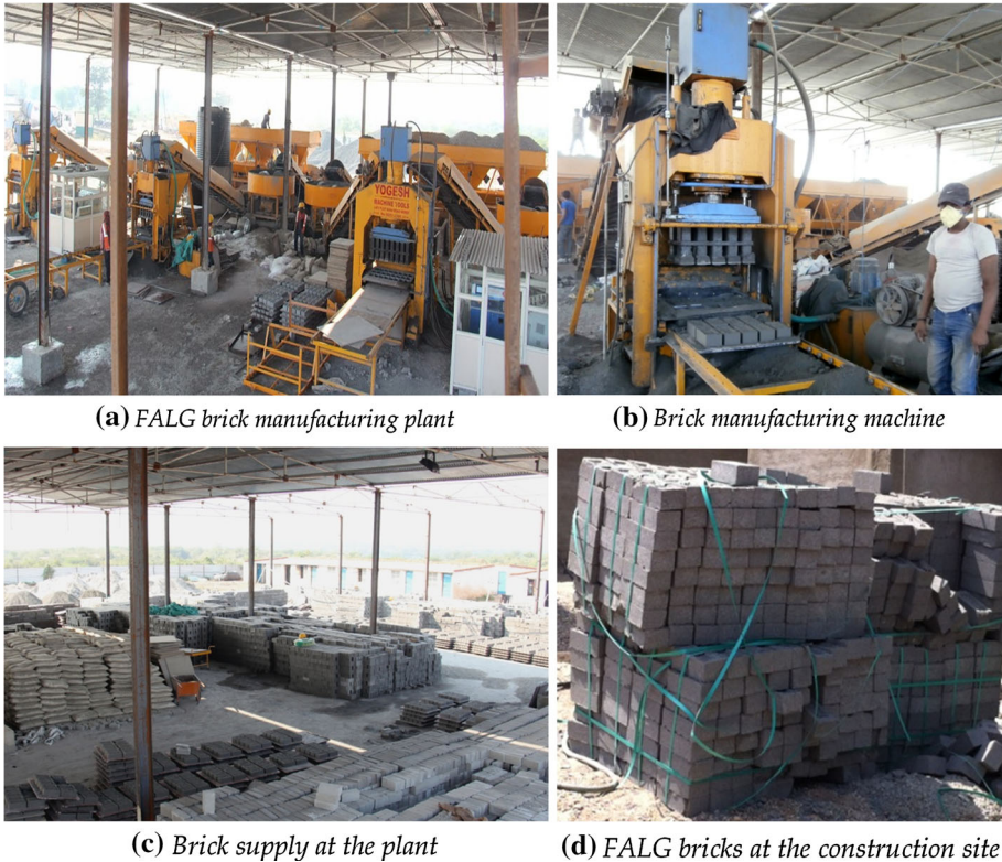
Fig. 59 Manufacturing process for FALG bricks at the IITGN campus construction site (Jain et al. 2015)
