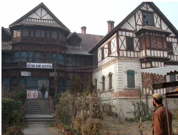
Fig. 14 Traditional construction is visible in this hospital in Kashmir, with upper storey of Dhajji Dewari and lower storey of masonry (photo: author)
