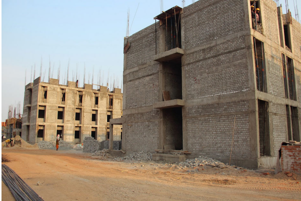
Fig. 56 Student hostels under construction, Feb 2014 (photo: S. Brzev)
