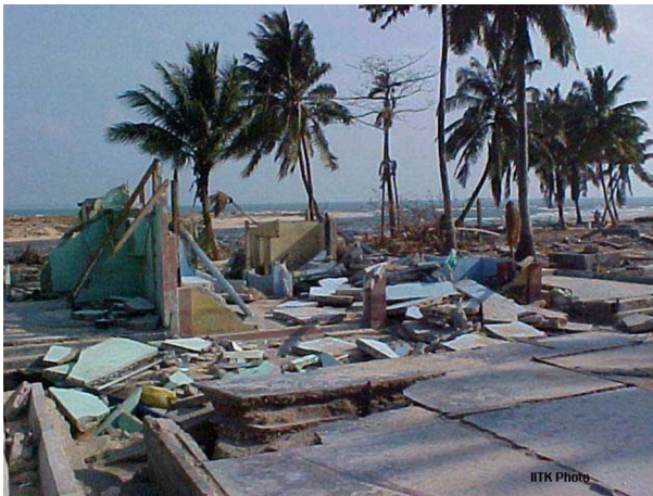
Fig. 50 Typical tsunami damage in coastal India (photo: C. V. R. Murty)
