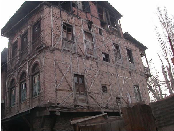
Fig. 13 Traditional Dhajji Dewari construction in Srinagar (photo: author)
