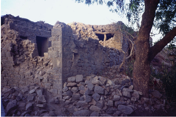
Fig. 39 Typical house construction with stone masonry in Marathwada (photo: S. Brzev)
