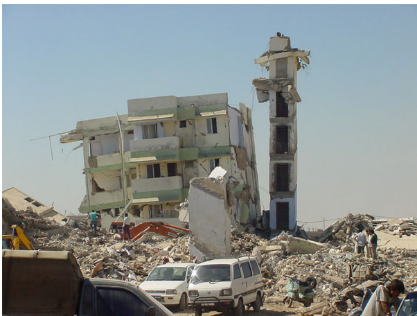
Fig. 6 Apartment collapse in 2001 Bhuj earthquake (photo: C. V. R. Murty)
