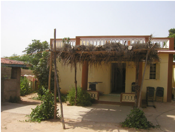
Fig. 48 Owner-rebuilt house in village of Sokhada (photo: C. V. R. Murty)
